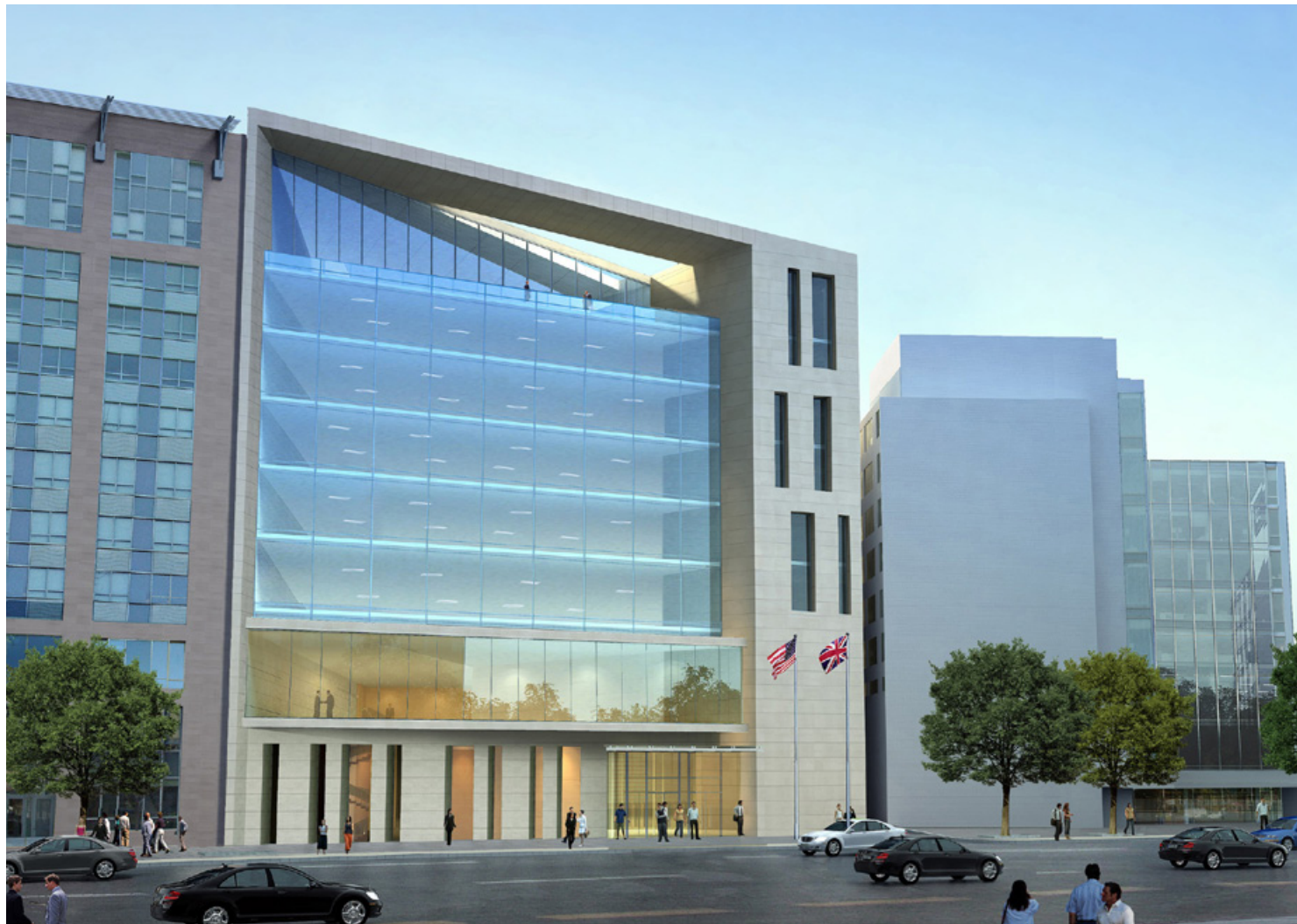
The new, 130,000 SF Center for Strategic & International Studies headquarters, designed by Hickok Cole Architects, will include a 3-story conference center and atrium, and 50,000 SF of underground parking. HITT Contracting is the general contractor. The project was designed to achieve LEED GOLD.
