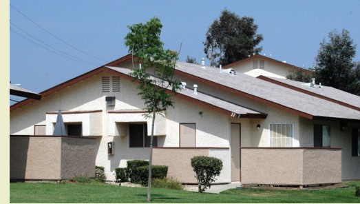
Highland's 108-unit Noble Creek project in Beaumont, California
