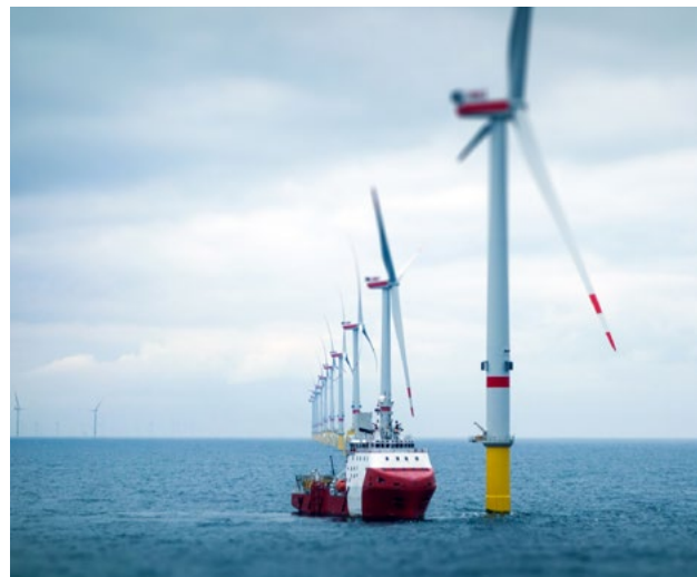
Figure 7: The Offshore Wind Farm Arkona, 35 km NE of the island of Ruegen, Germany
